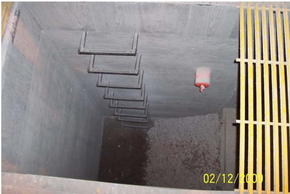
Photo 25- Sump with ladder and gravel slope installed.
