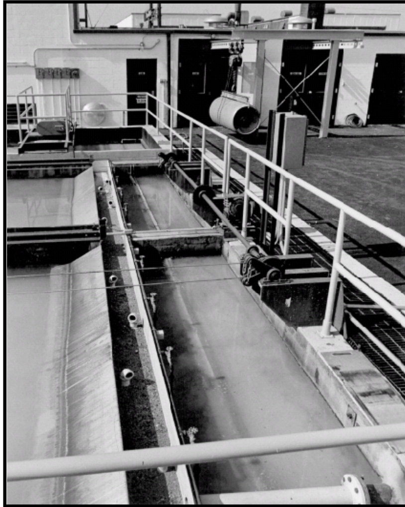
Photo 25 – Undated photo. View looking south from northwest corner of settling basins.
