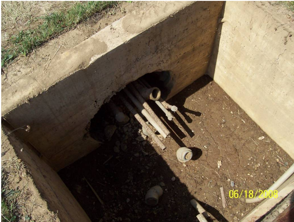
Photo 1 – View of pipe vault remaining from OWCA, looking southwest. Pipes remaining inside 24-inch dia. CMP.
