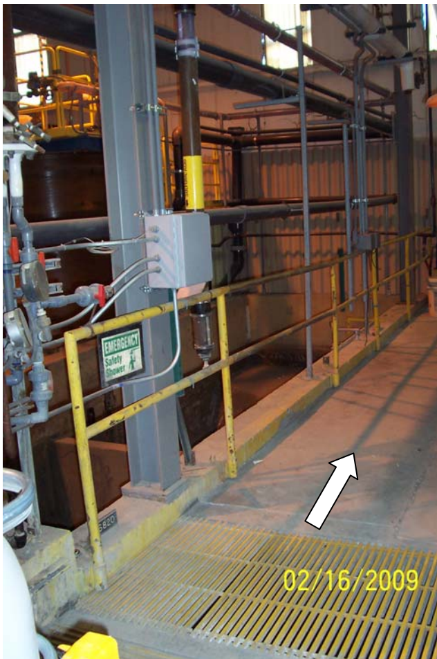
Photo 27 - Sump and trench remediation completed. North indicated by white arrow.
