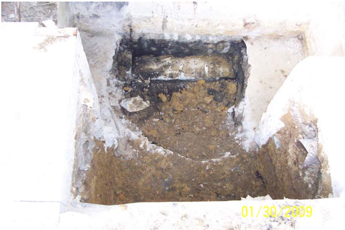
Photo 16 - Sump excavation. Impacted soil around footer of settling basin tanks. View looking west.
