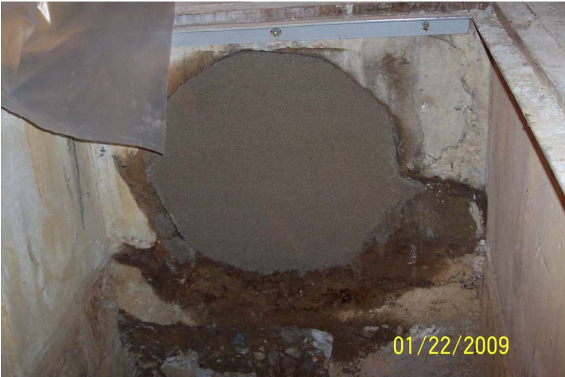
Photo 10 - 24" dia. corrugated pipe concreted after all pipes were removed.
