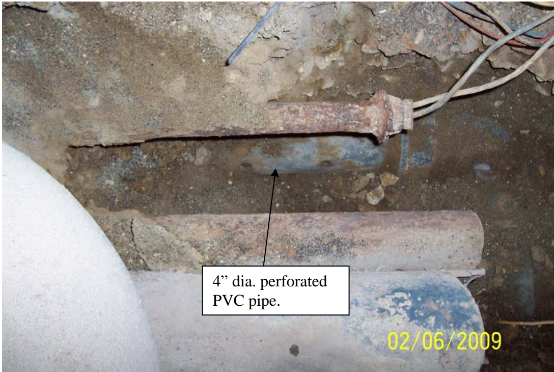
Photo 15 - 4" dia. PVC pipe continues in pipe trench by EQ. Note pipe is perforated.
