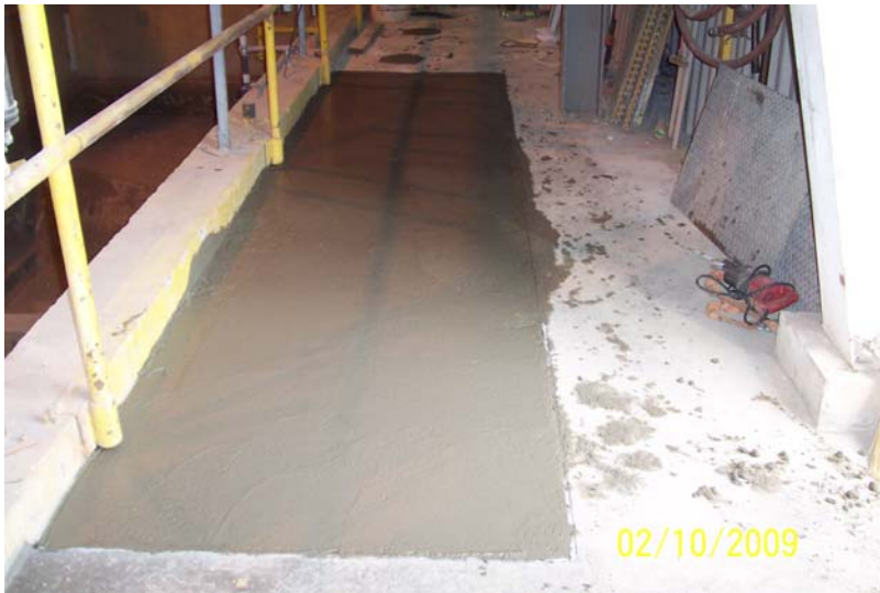
Photo 26 - Building 41 pipe trench concreted.
