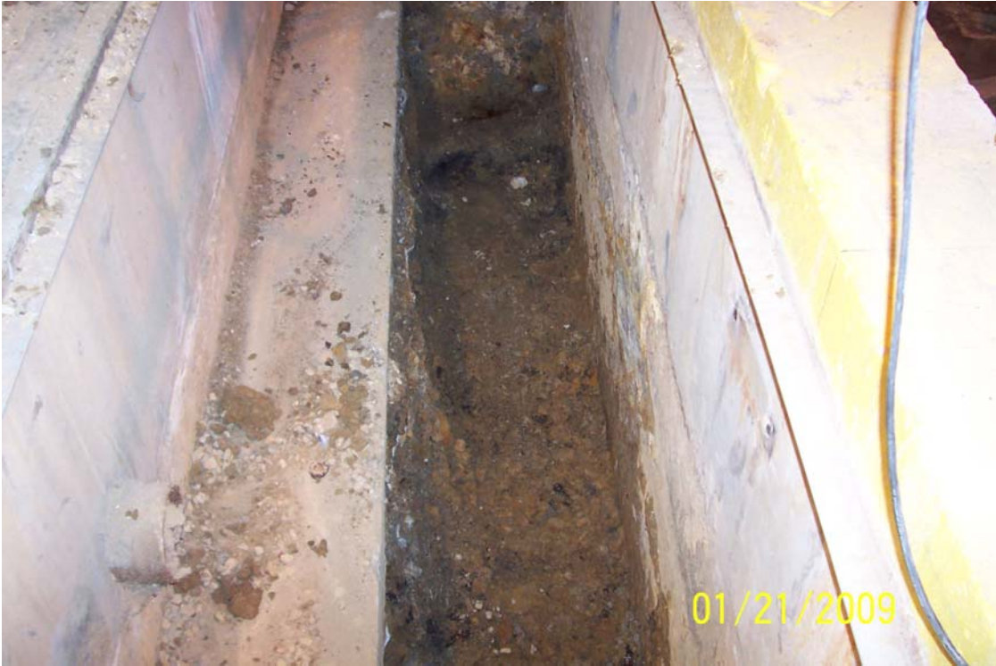
Photo 9 - Building 41 pipe trench looking south. Soil and pipes removed to depth.
