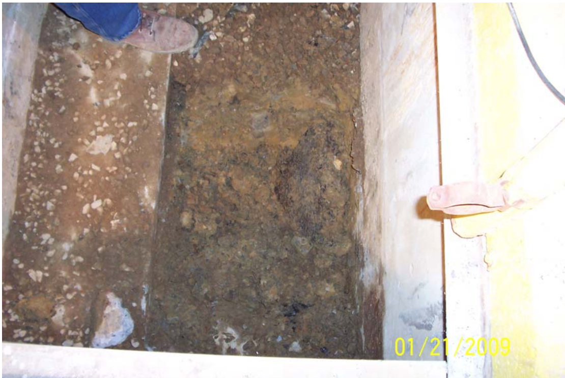
Photo 8 - Building 41 interior trench soil removal. View facing south.
