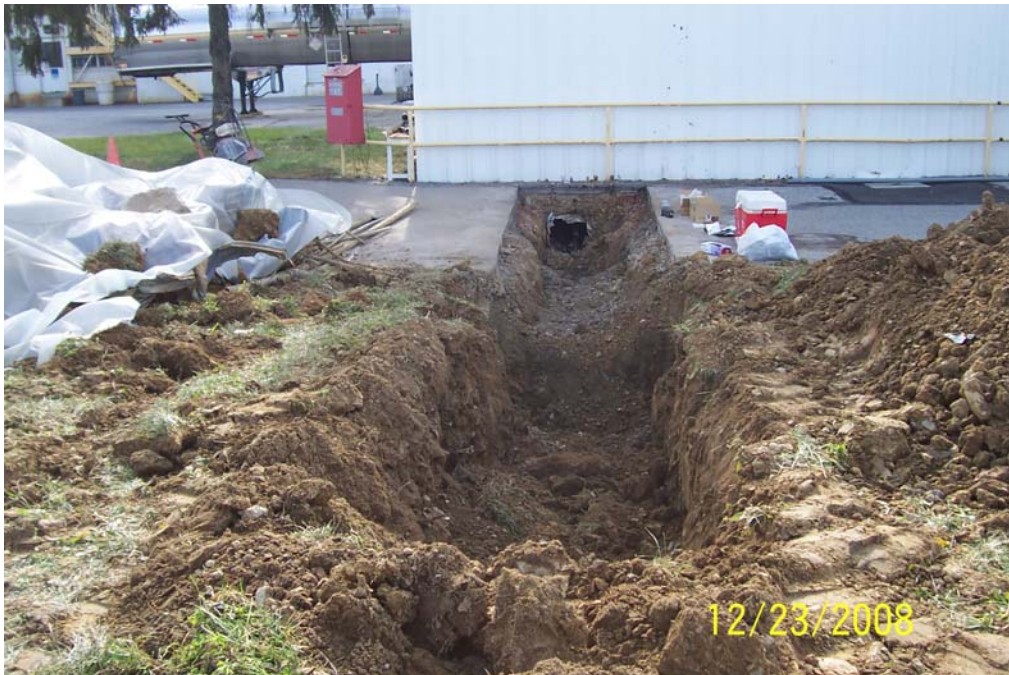
Photo 2 - Looking south at Building 41 outside trench and vault removal.
